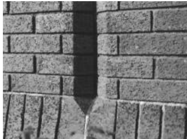
Accentuated Expansion Joint FIG. 9
