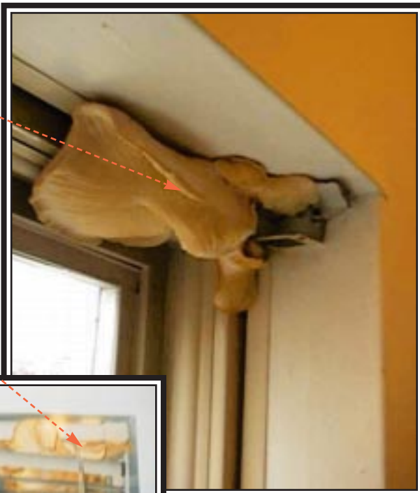
Mushroom/ fungi growing at window head due to elevated moisture levels
